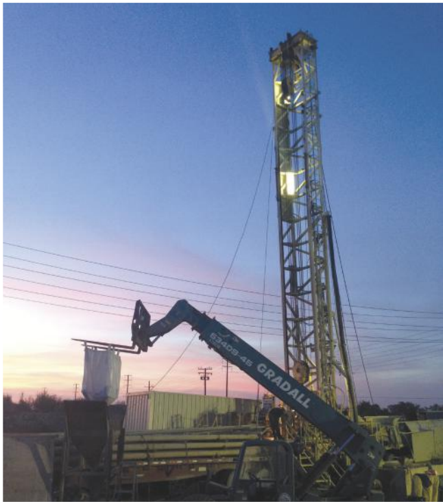
Above: In northern Claremont, a well is drilled to gain access to groundwater to supplement imported water supplies from northern California. Below: Water that is imported from northern California is distributed into spreading fields to percolate into groundwater basins for future use.
