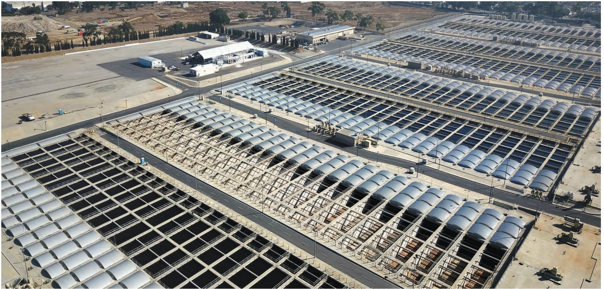
The Joint Water Pollution Control Plant (JWPCP) in Carson treats about 260 million gallons of wastewater per day, but most goes to the ocean. Pure Water Southern California, a joint project of the Los Angeles County Sanitation Districts and Metropolitan Water District of Southern California, would produce 150 million gallons per day (mgd) of purified water from the JWPCP for 15 million people upon completion in 2032.
