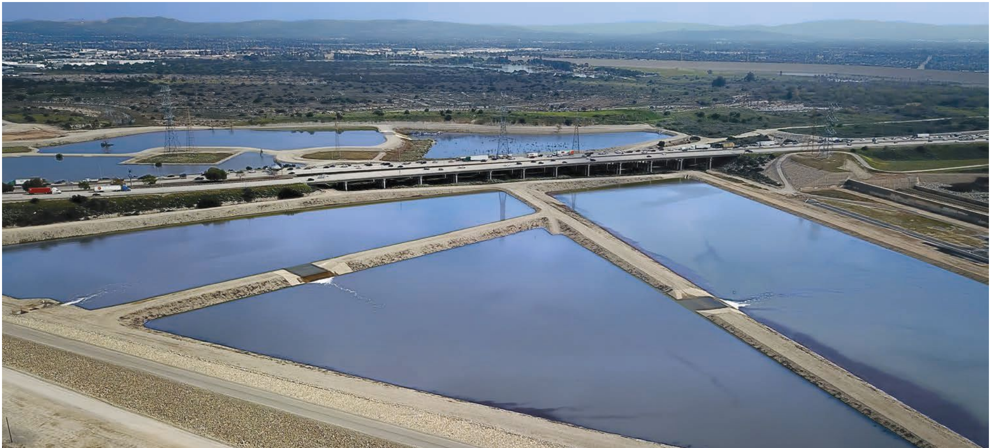
The Santa Fe Spreading Grounds, shown above, are operated and maintained by the Los Angeles County Flood Control District. The spreading grounds in Irwindale are designed to control flooding and conserve water through stormwater capture that recharges the Main San Gabriel groundwater basin.
