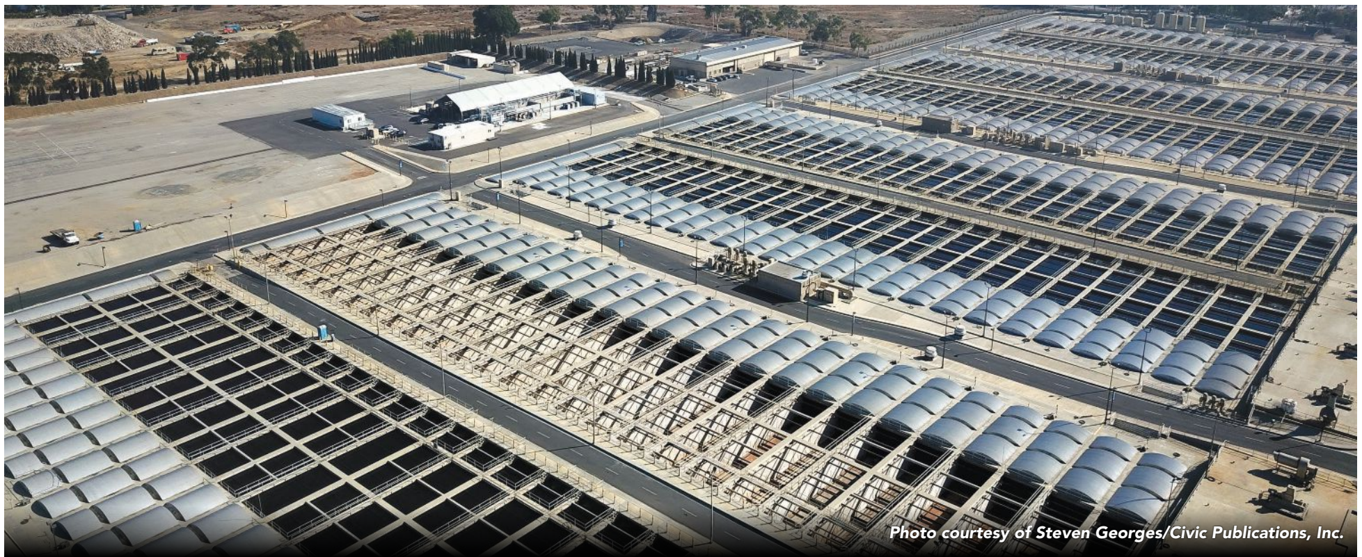
Above, the Joint Water Pollution Control Plant (JWPCP) in Carson treats about 260 million gallons of wastewater per day, but most goes to the ocean. Pure Water Southern California, a joint project of the Los Angeles County Sanitation Districts and Metropolitan Water District of Southern California, would produce 150 million gallons per day (mgd) of purified water from the JWPCP for 15 million people upon completion in 2032. At right, the Sites Reservoir Project will be situated on the west side of the Sacramento Valley, approximately 10 miles west of Maxwell in Glenn and Colusa Counties.
