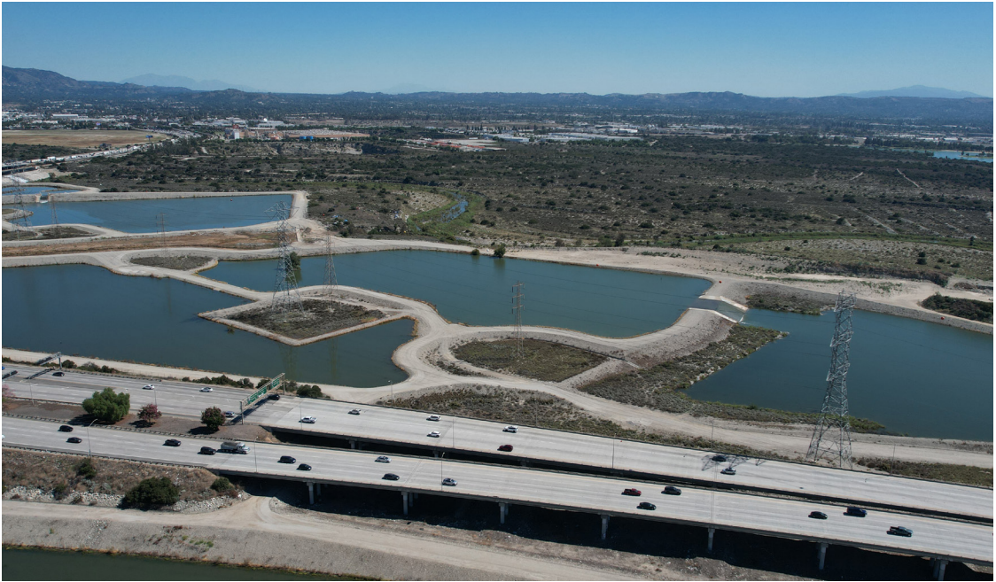
At far left and above is the Puente Valley Intermediate Zone Remedy Operating Unit, which is one of 32 active groundwater treatment facilities that are integral to the cleanup coordinated by the San Gabriel Basin Water Quality Authority. At left, the water percolates into the groundwater basin from the Santa Fe Spreading Grounds near the 210-605 freeway interchange.
