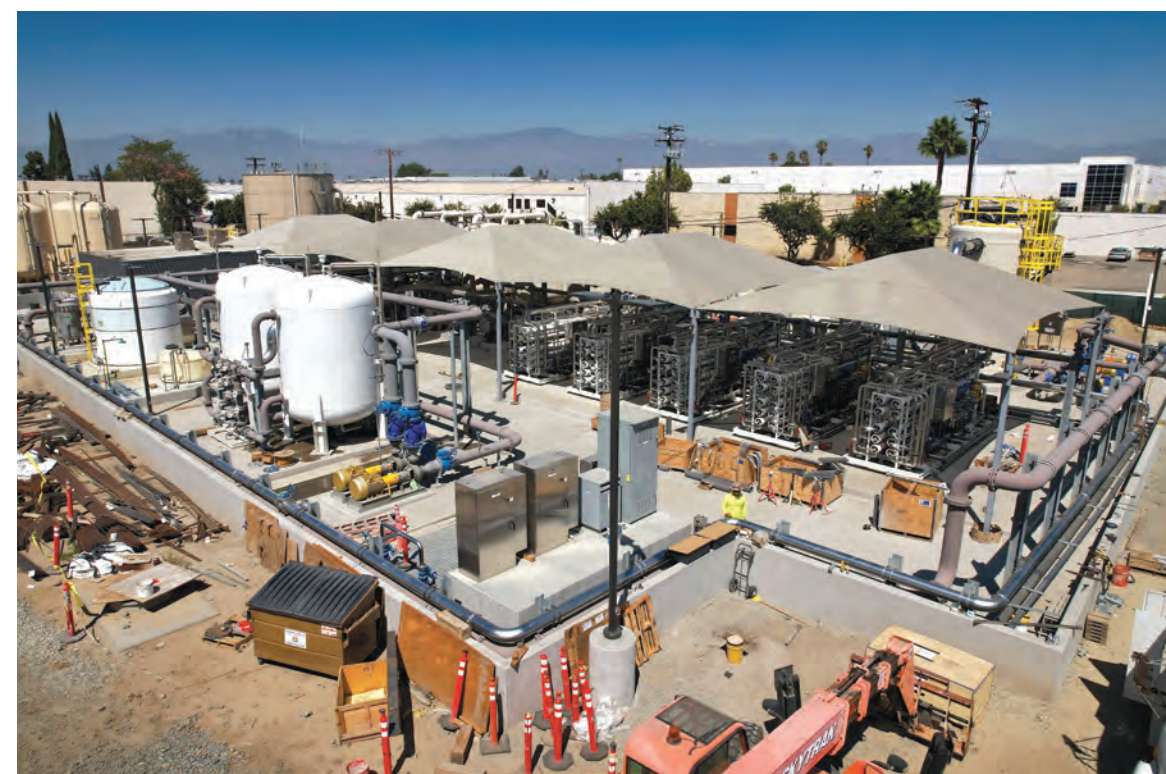
The Puente Valley Operable Unit Intermediate Zone Remedy is the first groundwater treatment facility in the basin to incorporate state-of-the-art Reverse Osmosis in its treatment process.
